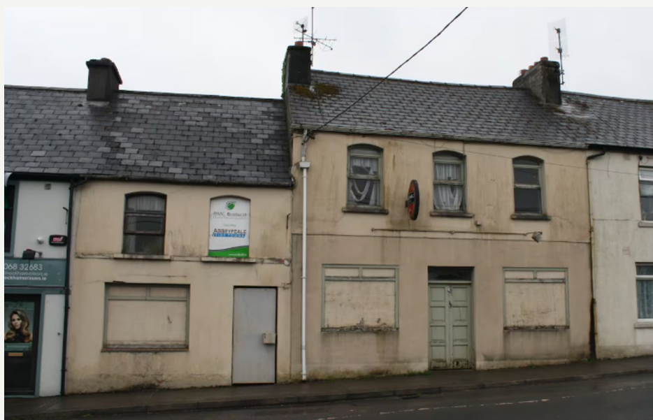
Bridge Bar Abbeyfeale Co. Limerick, before its conversion
