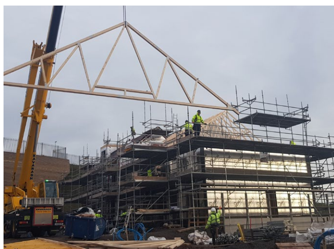
Timber Frame Construction
