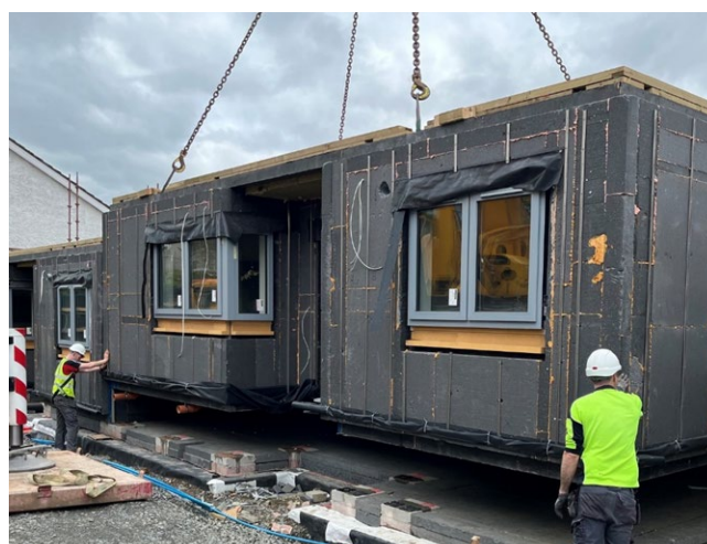
3-D Volumetric Units Installation
